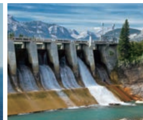
水力発電 Hydroelectric power generation
