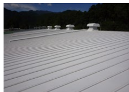
No. 2 Facility of Gifu Plant after application of the rooftop coating
