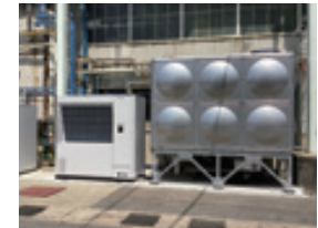
Installation of a heat pump
